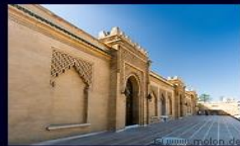
10 Red wall and gates
